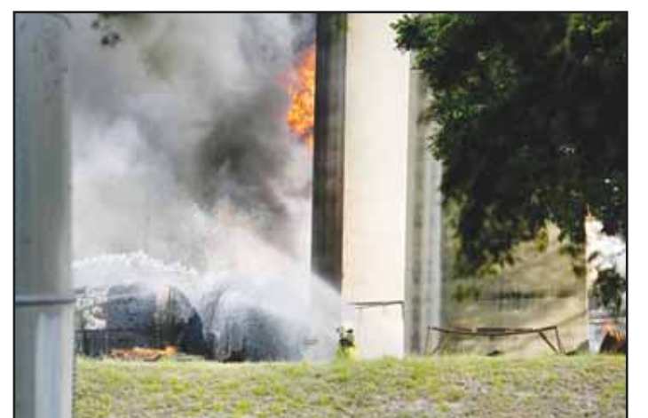
A firefighter sprays water on gas trucks that caught fire after several exploded under Las Americas Bridge next to the Panama Canal in Panama City, Panama on April 6. (AP)
