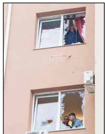
People remove broken glass from their windows after a Russian strike on residential neighbourhood in Kriukivshchyna, Kyiv region, Ukraine, on April 3. (AP)
