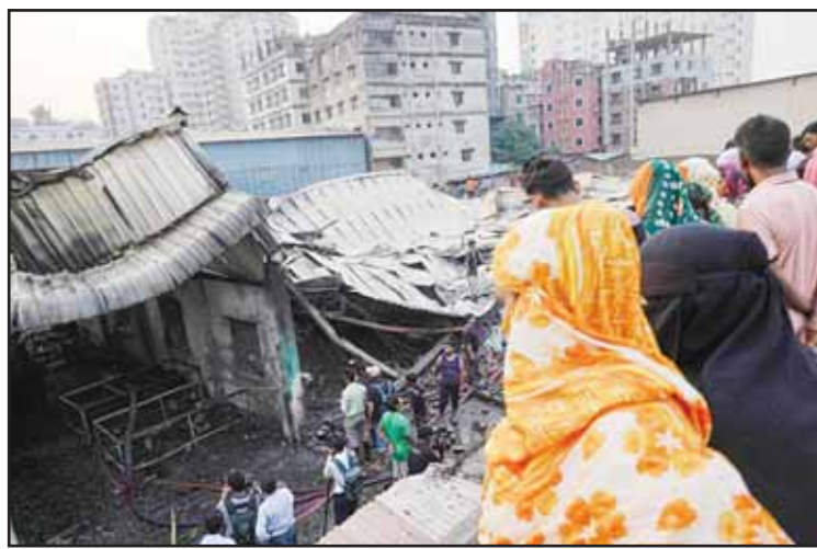
People look at the charred remains of a gas-lighter manufacturing factory in Keraniganj on the outskirts of Dhaka, Bangladesh on April 4. (AP)
