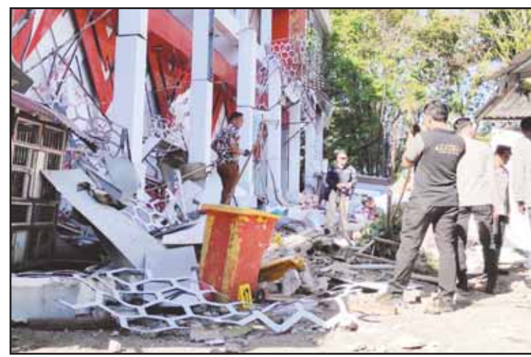
Police officers inspect a damaged building following an earthquake in Manado, North Sulawesi, Indonesia on April 2. (AP)
