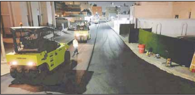
Road maintenance continues in Al-Ardhiya area.
