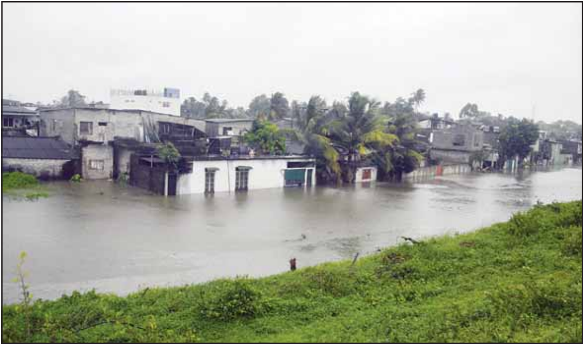
This photo taken on Nov. 28, 2025 shows submerged houses after heavy rains in Kolonnawa, Sri Lanka. (Xinhua)
