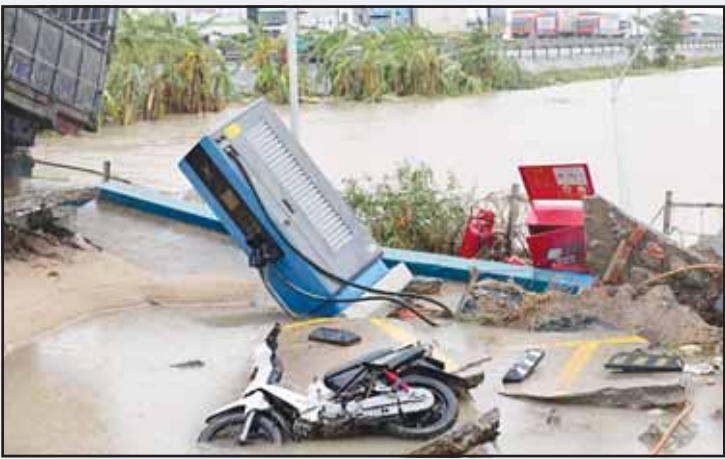
This photo taken on Nov 22, 2025 shows a section of national highway damaged by flood in Dak Lak Province, Vietnam. (Xinhua)
