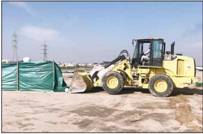
A Municipality bulldozer dismantles tents set up illegally in the desert. Municipality photo
