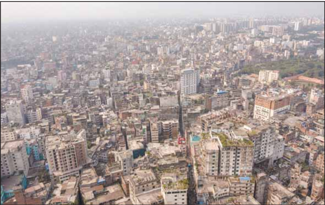
A general aerial view of an old city where roofs and walls collapsed after an earthquake in Dhaka, Bangladesh on Nov 21. (AP)
