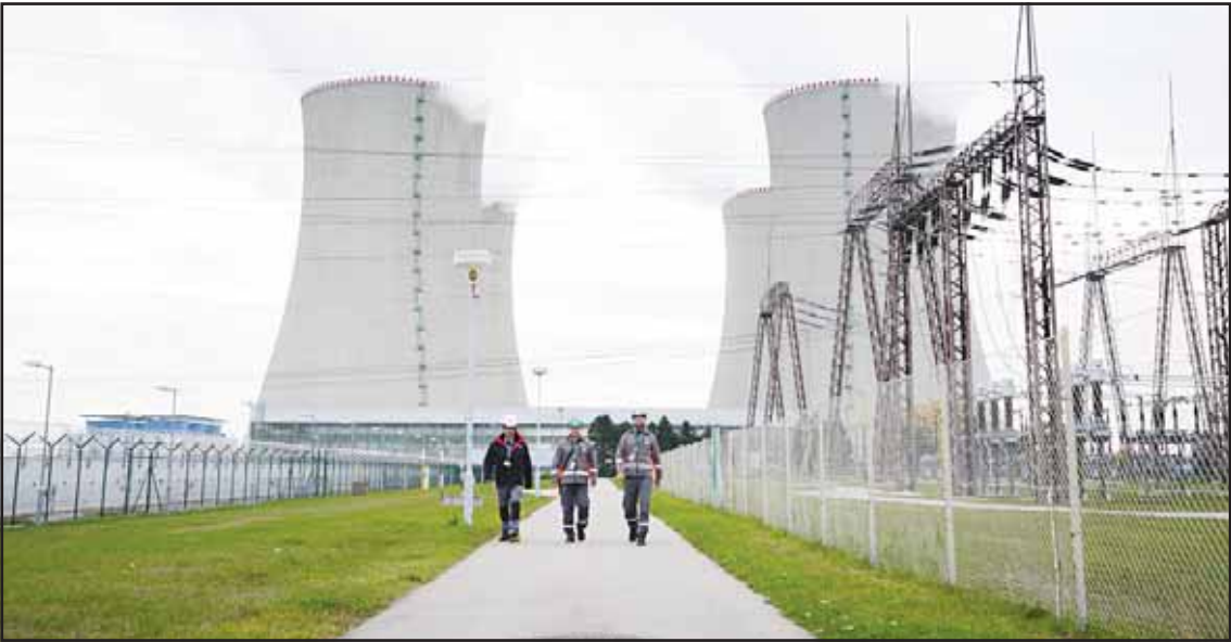
Workers walk past cooling towers of the Dukovany nuclear power plant in Dukovany, Czech Republic, Oct. 21, 2025. (AP)
