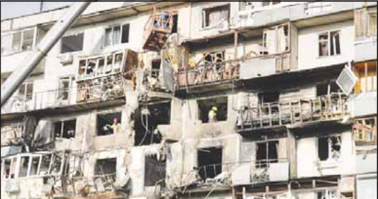
Rescuers work on the scene of a building damaged after a Russian attack in Kyiv, Ukraine, on Nov 14. (AP)
