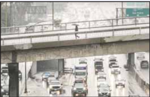
A pedestrian with an umbrella walks on a bridge over the rain-soaked 110 Freeway in Los Angeles on Nov 14. (AP)
