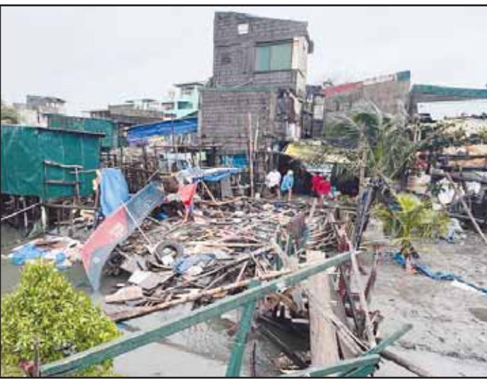
Residents stand beside a damaged house and toppled bridge due to Typhoon Fung-wong along a coastal village on Nov 10, in Navotas, Philippines. (AP)
