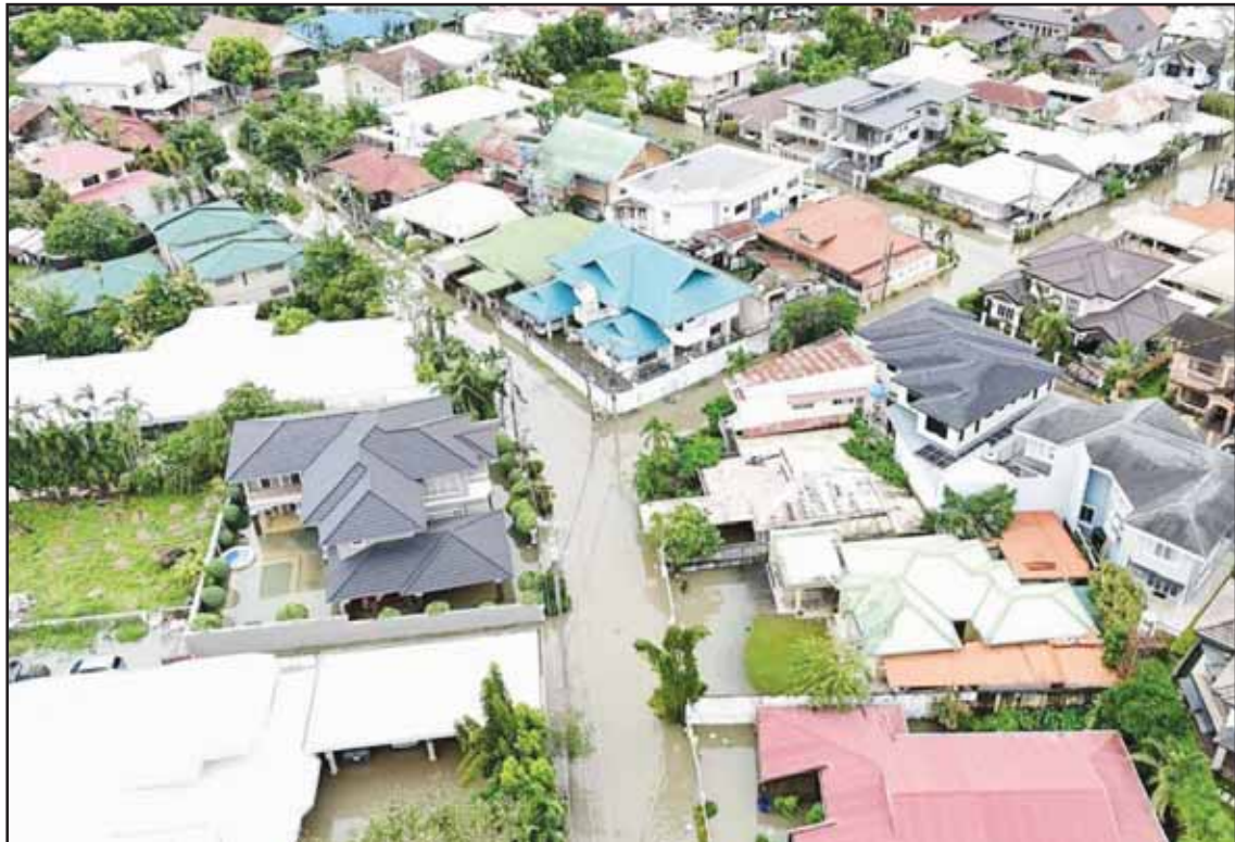
Residential areas are flooded by Typhoon Kalmaegi as it affects Cebu City, central Philippines on Nov 4. (AP)
