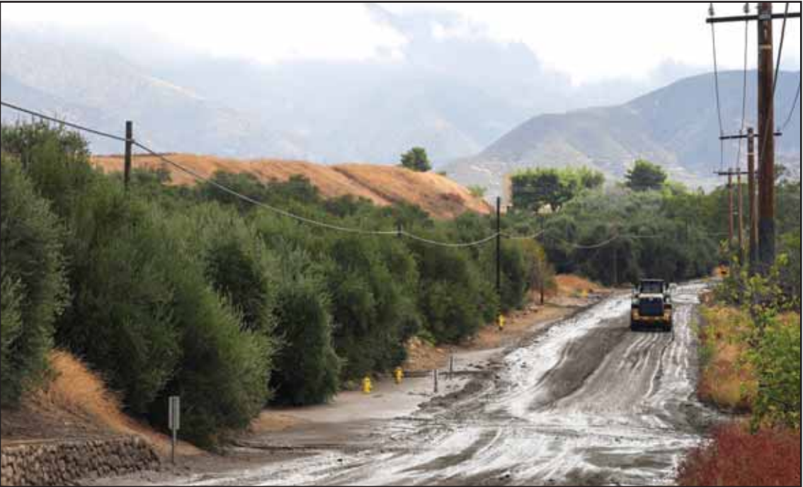
Workers clean up the damage caused by mudslides after storms in Yucaipa, Calif., Friday, Sept. 19, 2025. (AP)
