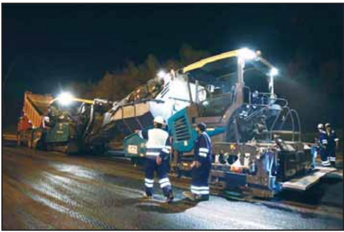
Asphalt is laid on Khalaf Al-Ahmar Road in Sulaibikhat.
