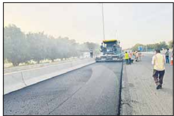
Road paving under progress in Farwaniya. Al-Seyassah photo
