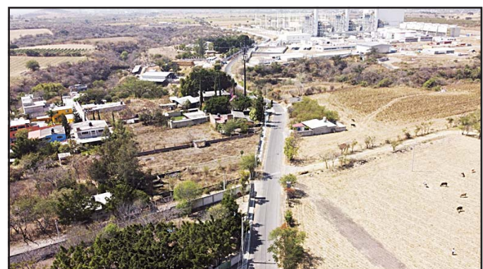
In this file photo, a power generation plant stands idle near Huexca, Morelos state, Mexico. A constitutional reform presented by President Andrés Manuel López Obrador would cancel contracts under which some private power generating plants sell power into the national grid. (AP)
