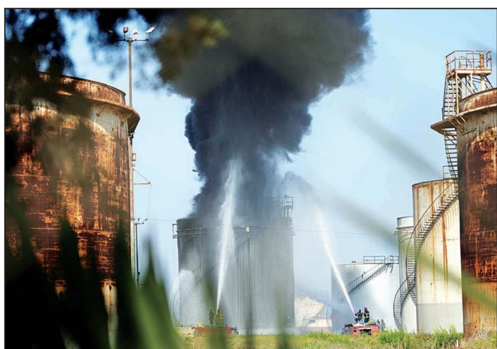
Firefighters work to extinguish a fire in an oil facility in the southern town of Zahrani, south of the port city of Sidon, Lebanon, Monday, Oct. 11. A huge fire broke out at an oil facility in southern Lebanon's coastal town of Zahrani, but the cause was not immediately known. Energy Minister Walid Fayad said the fire broke out when workers were transferring gasoline from one storage tank to another in the coastal town of Zahrani. He said nearly 250,000 liters (66,000 gallons) of gasoline were burnt during the blaze, which lasted more than three hours. No one was reported hurt. The fire came as cash-strapped Lebanon struggles through a serious power crisis partly due to severe shortages in fuel that have resulted in electricity cuts lasting up to 22 hours a day. (AP)
