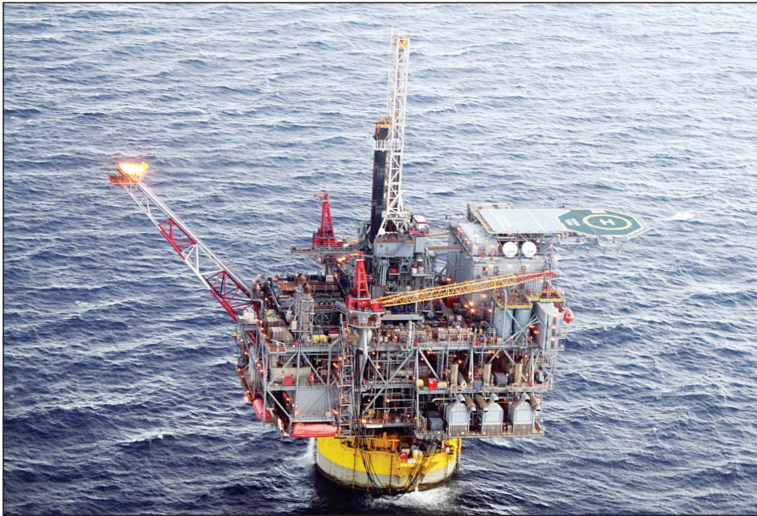
This file photo, shows the Perdido oil platform located about 200 miles south of Galveston, Texas, in the Gulf of Mexico. The US is holding a large oil and gas lease sale in the Gulf of Mexico after a federal judge in a lawsuit brought by Republican states rejected a suspension of fossil fuel sales that Biden imposed when he took office. (AP)
