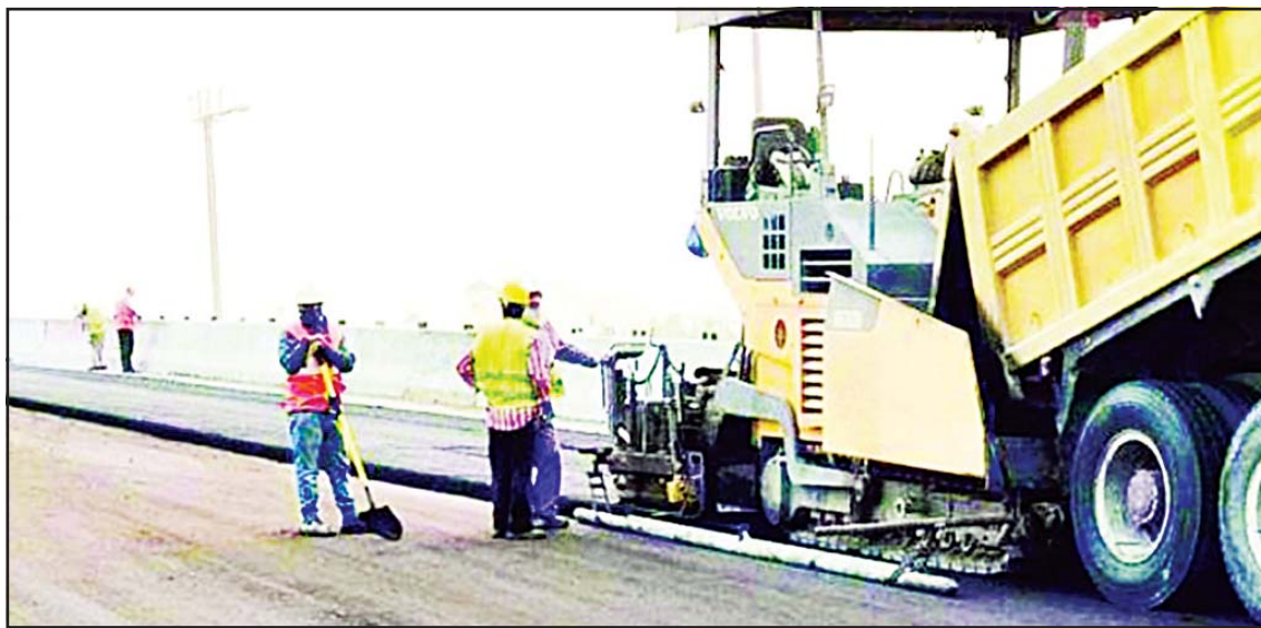
Asphalt laying in progress in one of the areas.
