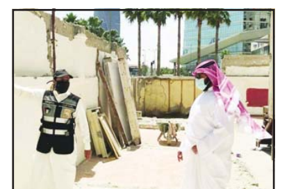
Capital Governor Sheikh Talal supervising the demolitions.
