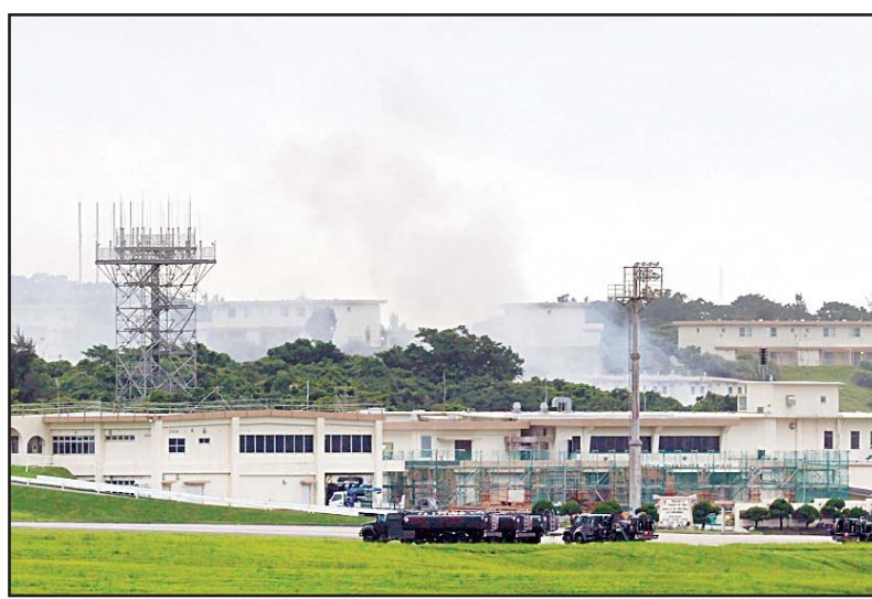
Smoke rises from the 18th Wing Hazardous Materials Pharmacy building at Kadena Air Base during a fire on Okinawa island, Japan, Monday morning, June 22. Cause of fire is unknown, no injuries are reported. (AP)
