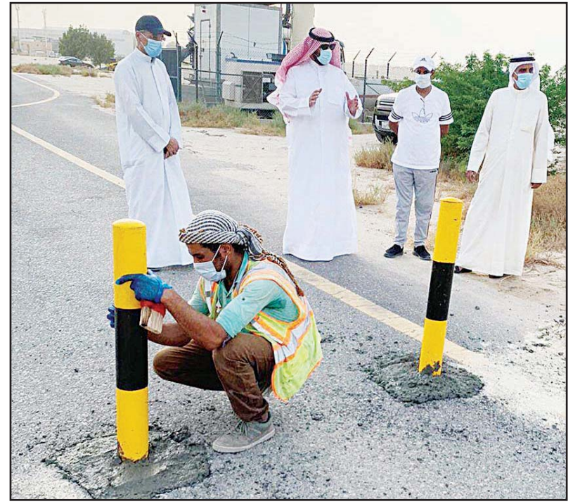
Iron barriers being installed on Sulaibikhat walkway.
