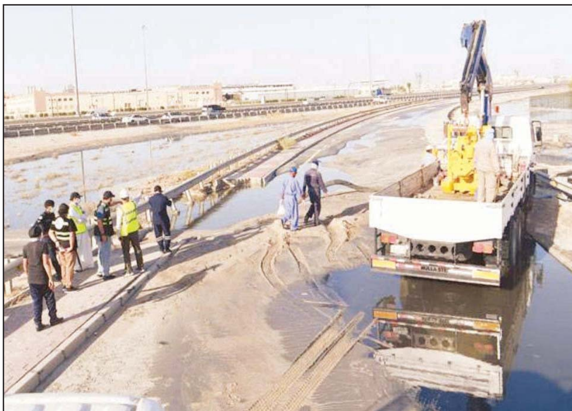
Work on cracked pipe ongoing.
