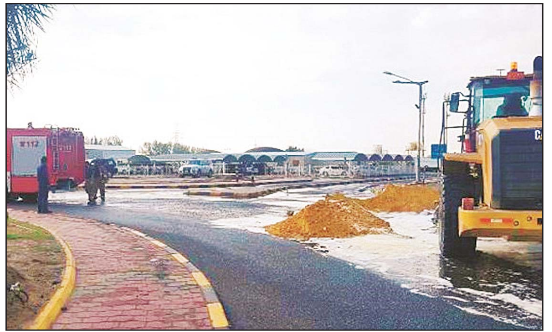
Sand is dumped on the hazardous material spilled on the road.
