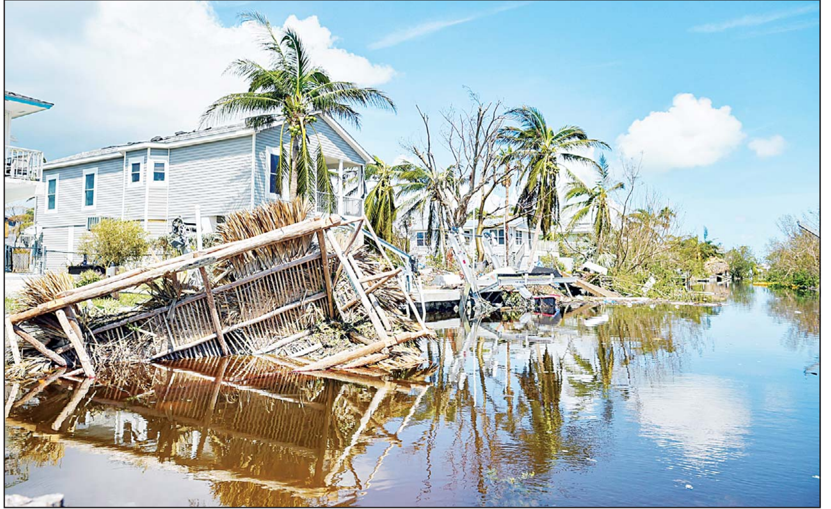
Damaged homes near Marathon, Florida on Sept 12, after Hurricane Irma. Florida is cleaning up and embarking on rebuilding from Hurricane Irma, one of the most destructive hurricanes in its history. (AP)
